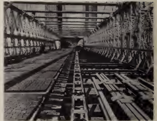
After removal of tracks, new steel stringers were laid.
